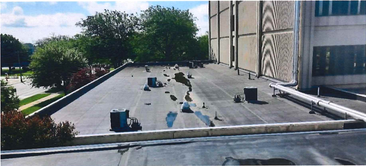
Figure 6: County Office Building Roof
