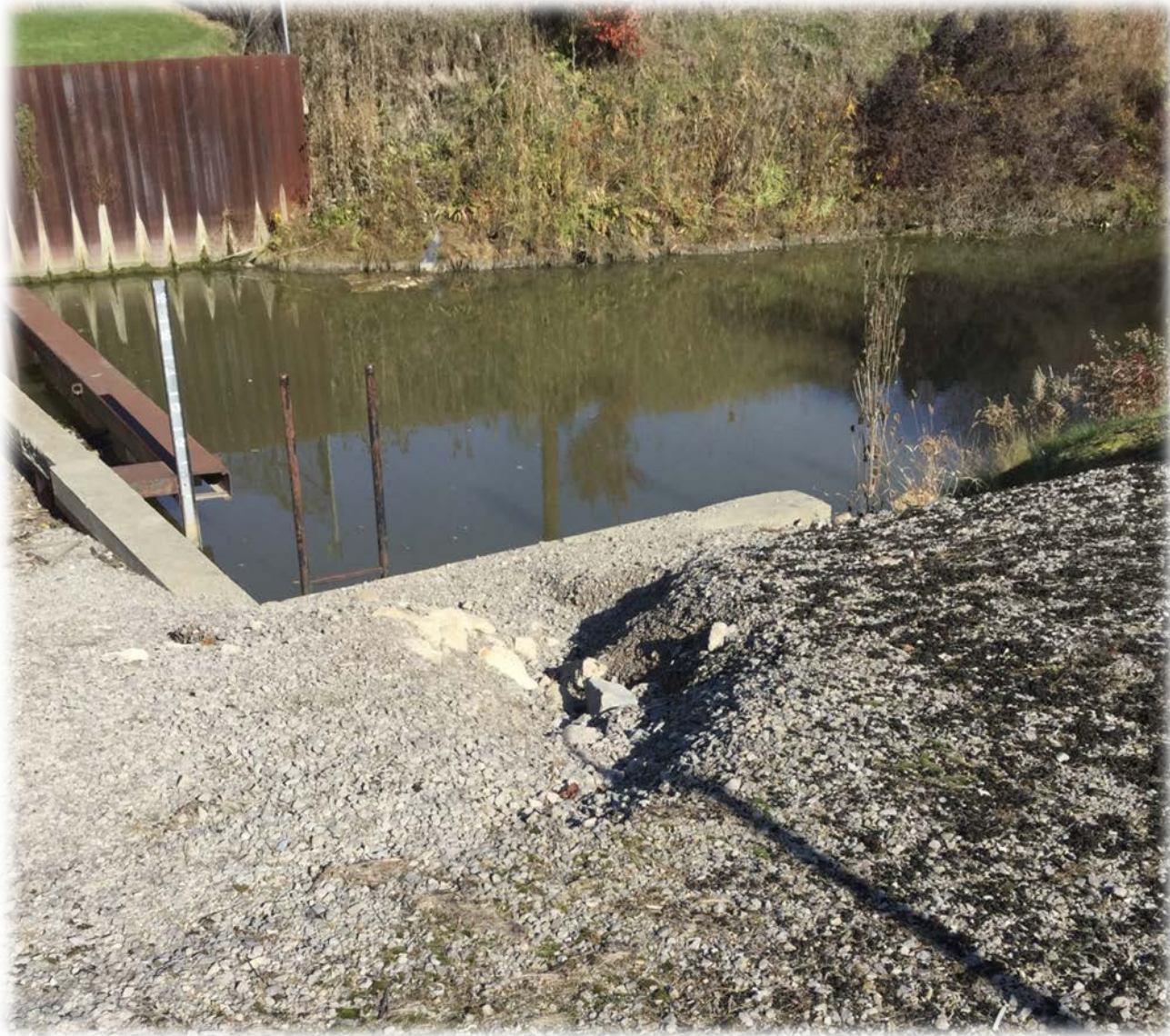
Soil Erosion Near Trash Pit
