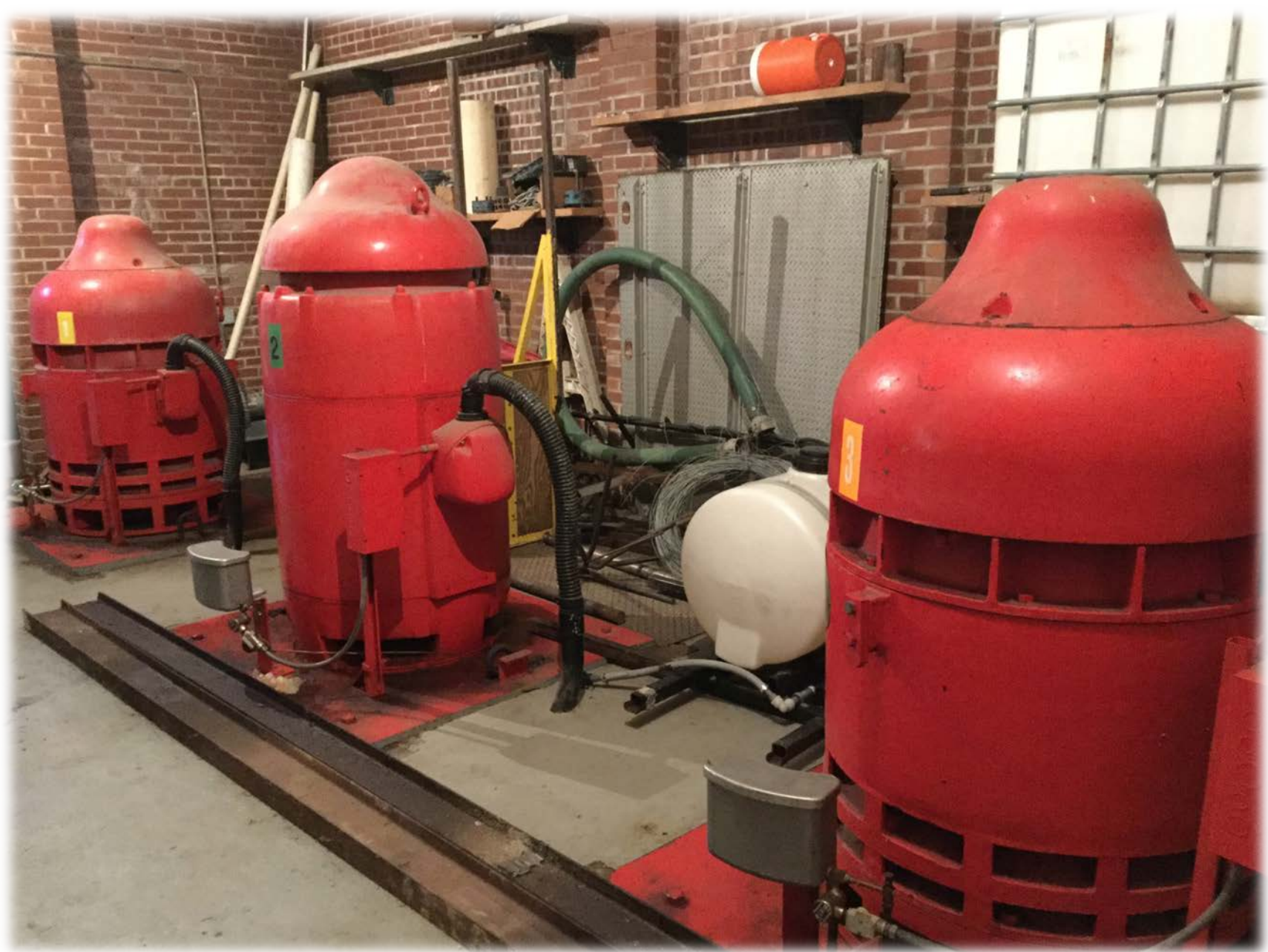
Pumps 1 & 3 are original. Pump 2 is newer model.
