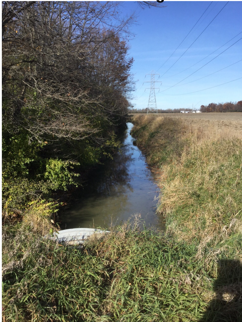
Looking Downstream (North) from Farm Crossing
