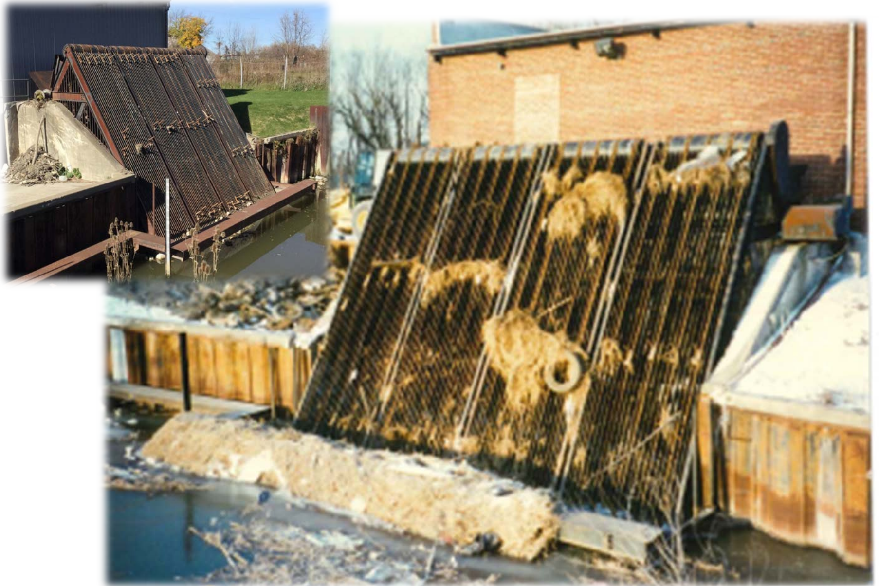
Trash Rack – Installed 1985
