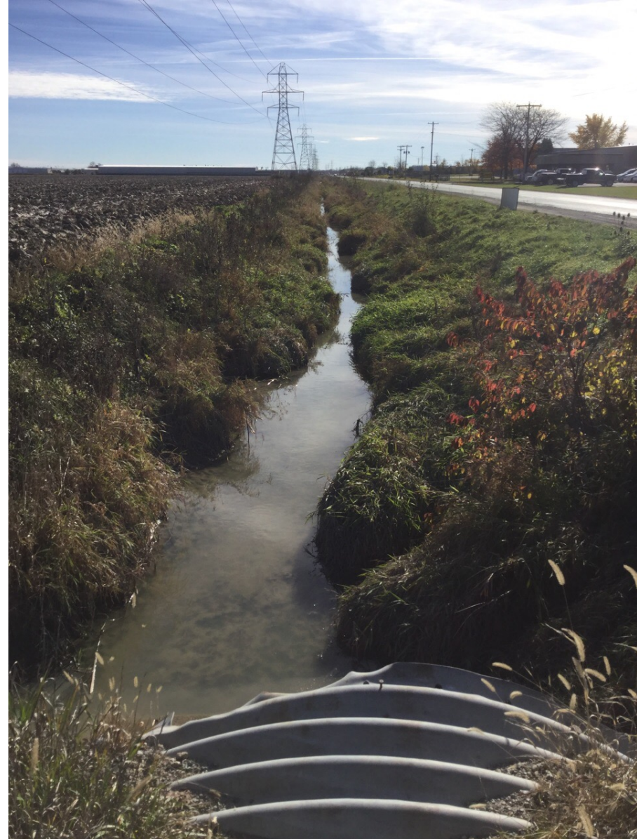
Looking Upstream (South) from Hack Road
