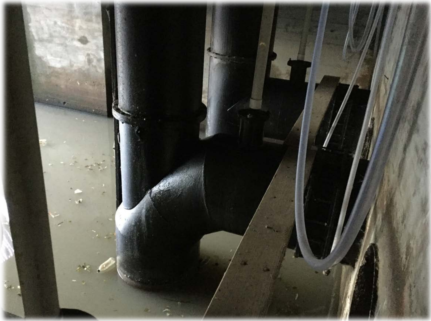
Wet Well – Problems with pumps freezing, confined space entry required to access, and no safety railings
