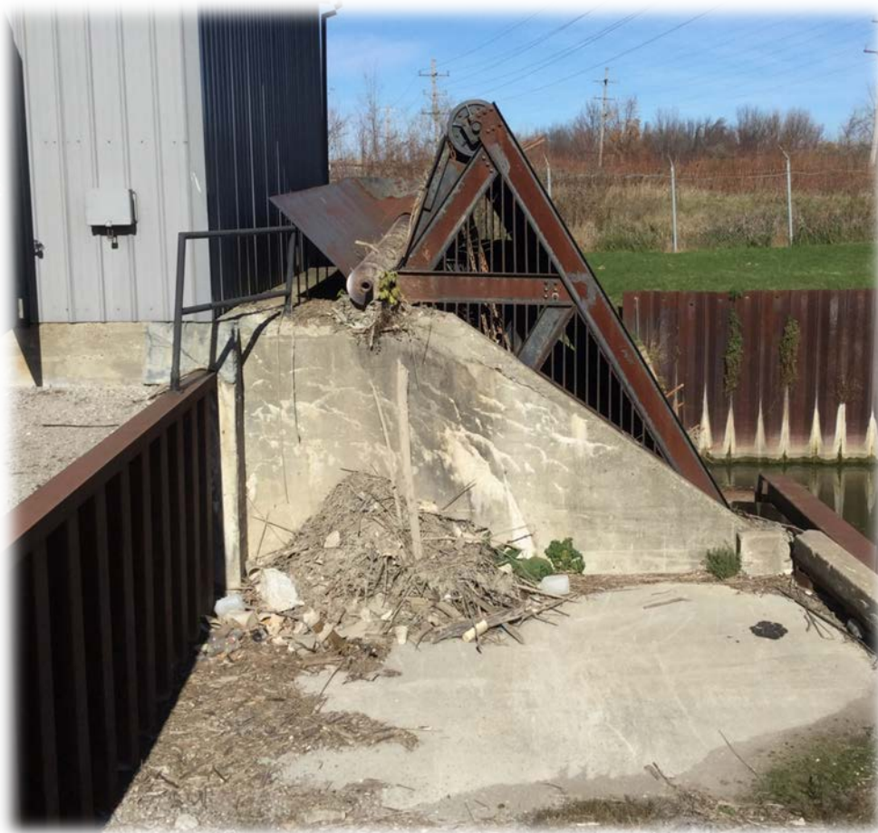
Trash Rack: Debris Pit Costly to remove debris. Trash must be separated, loaded into a dump truck, and hauled away.
