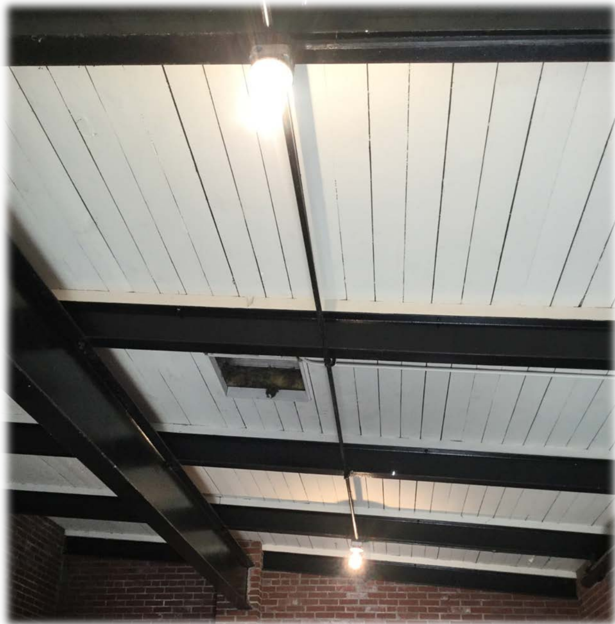
Pump Station Interior Lighting
