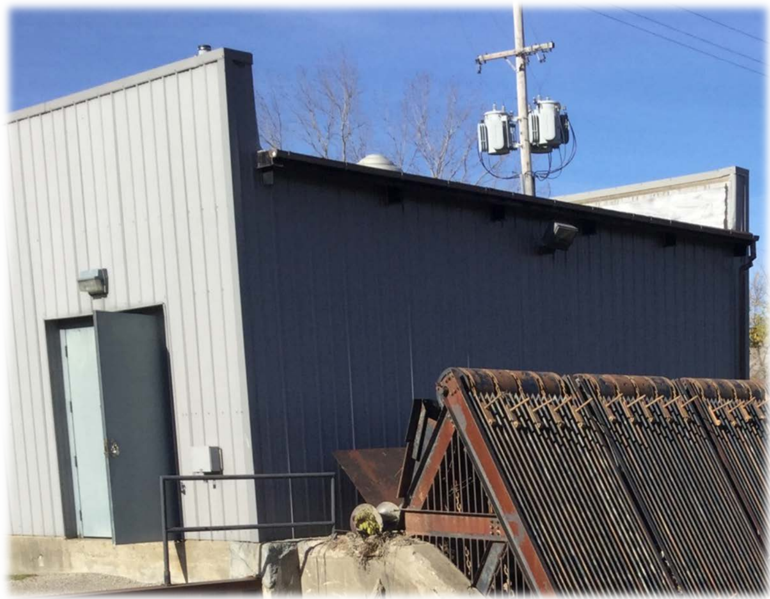
Pump Station Exterior Lighting
