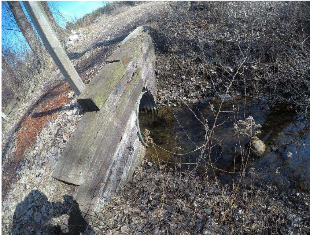
Crossing #32 Hatfield to be replaced with CMP
