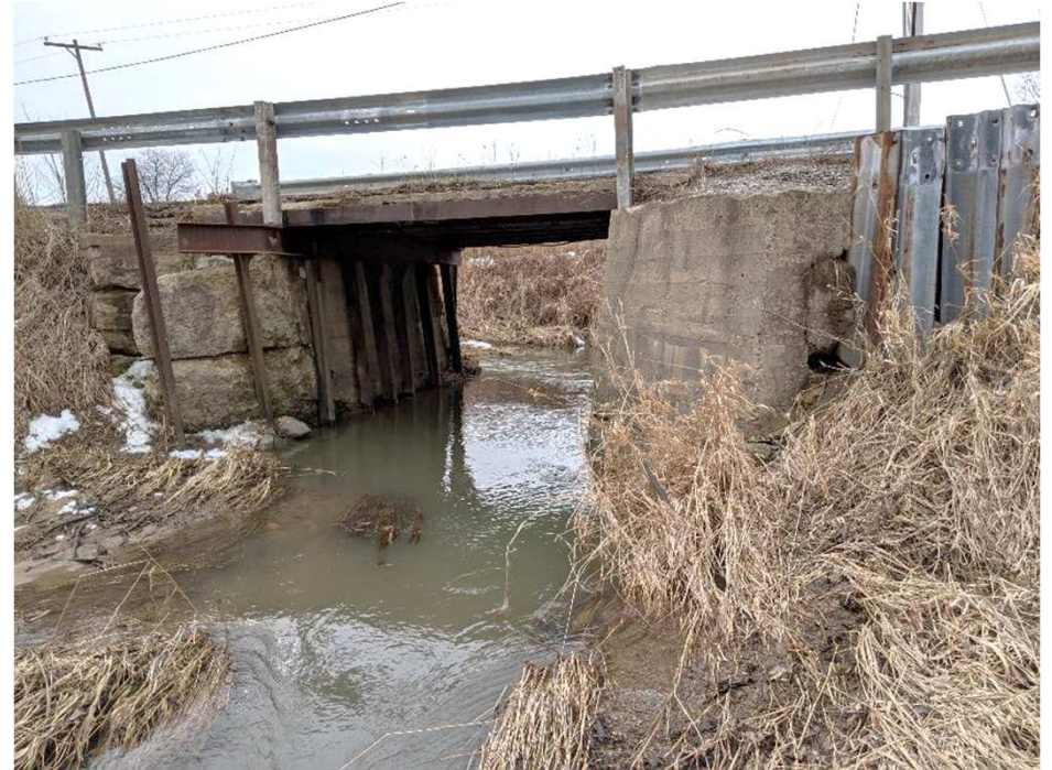
Crossing #4 Raucholz Rd. to be replaced with CMP Culvert
