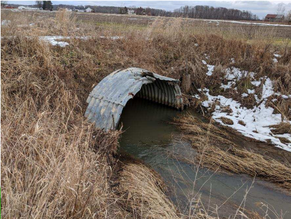
Crossing #3 Zelinko to be removed/relocated because of drain realignment
