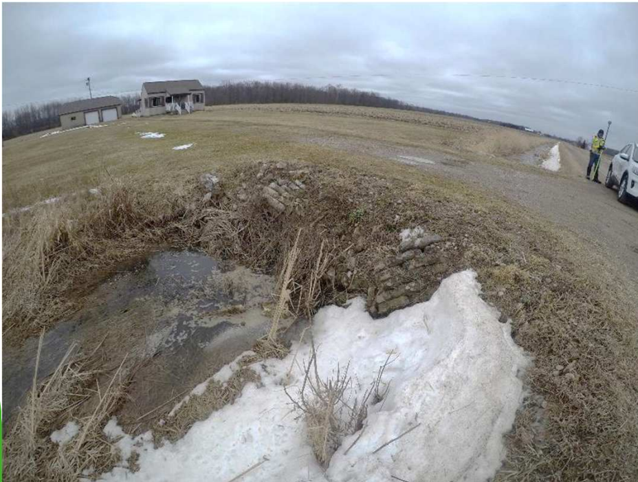
Crossing #24 Slocum to be replaced with CMP
