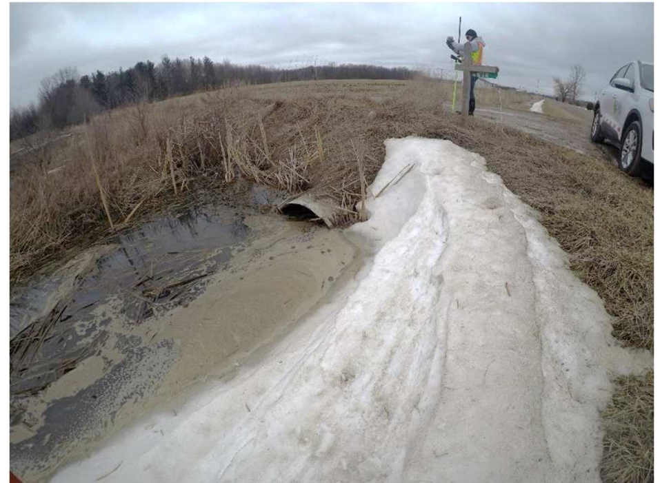
Crossing #25 Walter to be replaced and lowered
